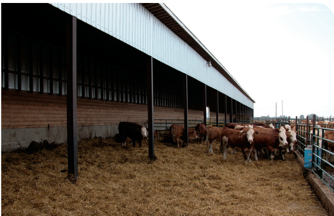
Figure 24. Exterior of an open front beef barn with yard.
