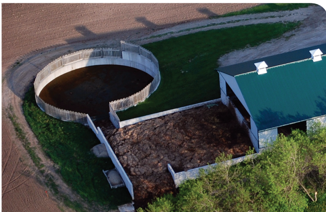
Figure 38. Uncovered liquid runoff storage (L1).
