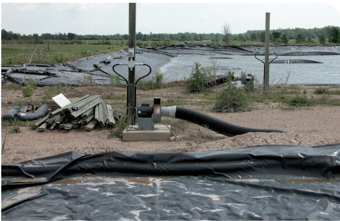
Figure 36. Tight-fitting negative pressure tarp for liquid earthen manure storage (V6).
