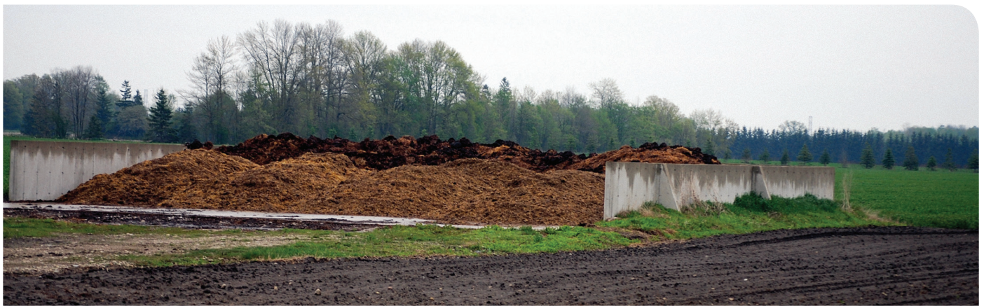
Figure 33. An outdoor, uncovered solid manure storage (V3).
