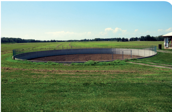
Figure 41. In-ground, uncovered, vertical wall liquid manure storage (M1).
