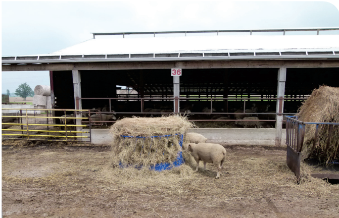
Figure 22. Exterior of a sheep barn and yard.
