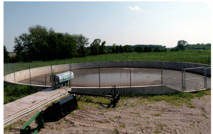
Figure 42. An above-grade, uncovered, vertical wall liquid manure storage and clean-out access ramp (M1).
