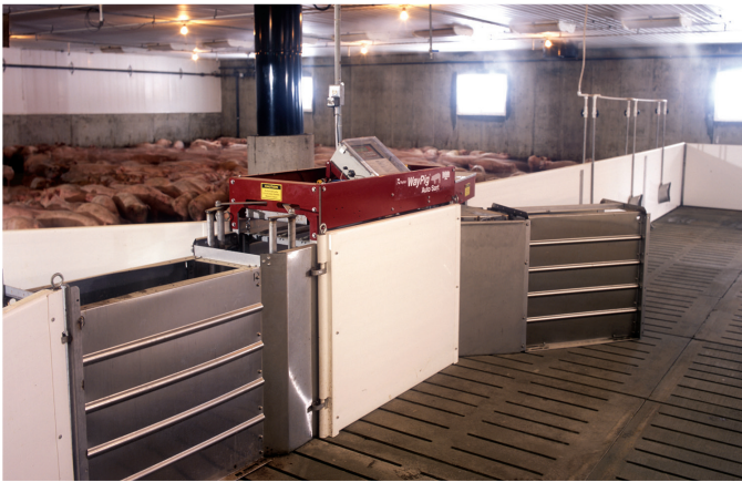
Figure 35. Slatted floor of barn for liquid manure storage under the barn (V5).
